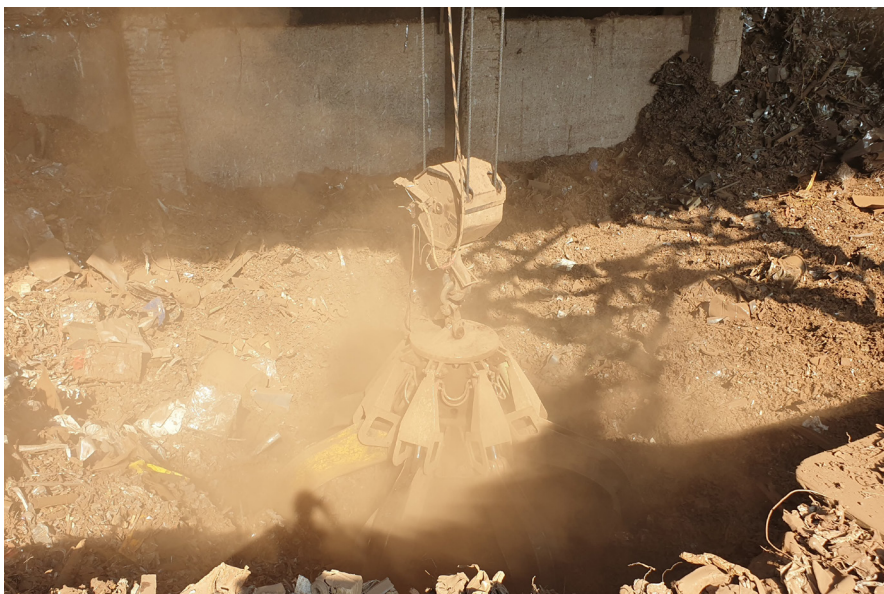
Tracking of movement of the overhead crane in operation.
