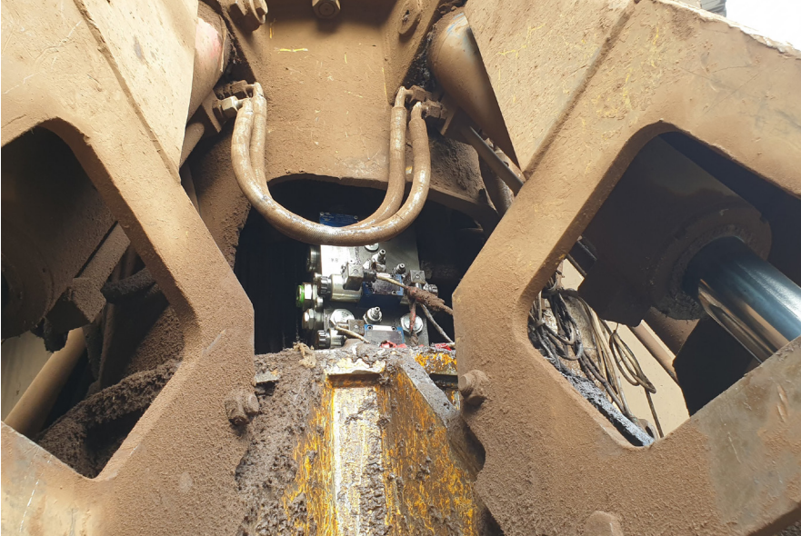
Detail of the open/closed switch of the crane.
